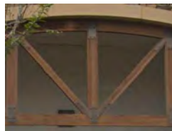
10 WOOD ARCHWAY BROWN TEAK WOOD REF. MATCH EXISTING SHIPPING CENTER REF. COLOR CUSTOM BROWN SEE 3/A-400
